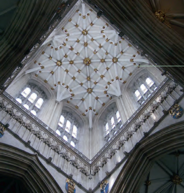
Interior view of the tower of York Minster cathedral
